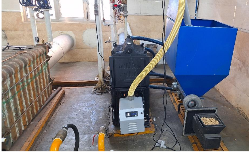
Figure 8- Burner & Boiler Installation
